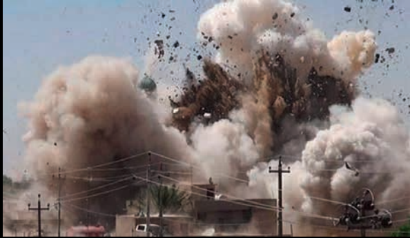
Destruction of Mar Gorgees Church, Mosul, Iraq
